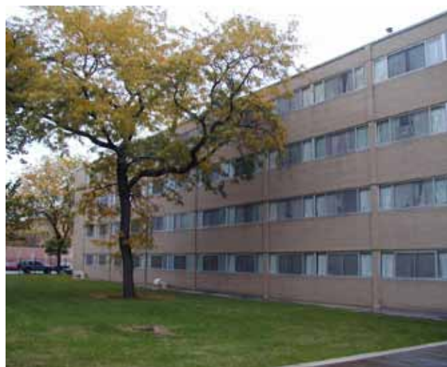
McCormick Student Residence
