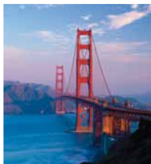
Golden Gate bridge
