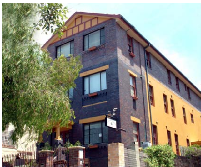
Bennett Street Hostel
