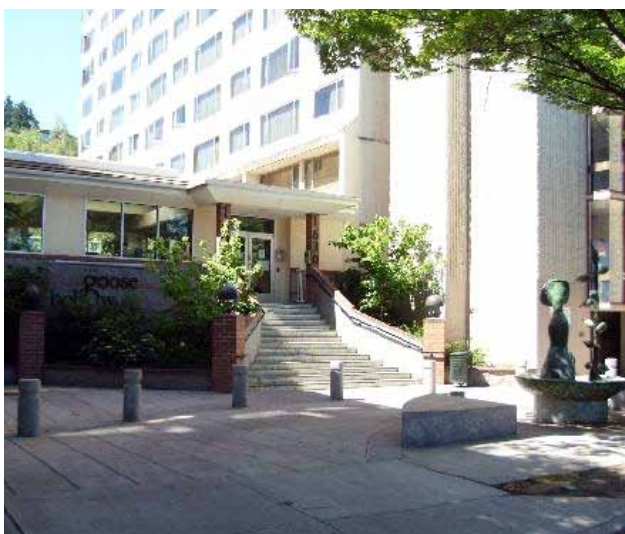
Goose Hollow Tower
