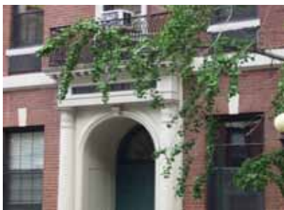
Front entrance of the residence
